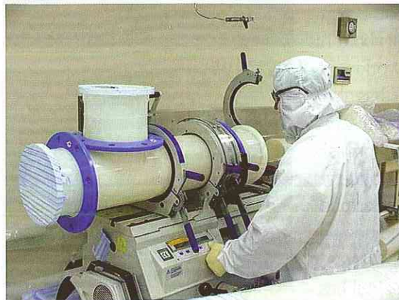
JBH Clean Room
